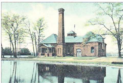
The Pumping Station
